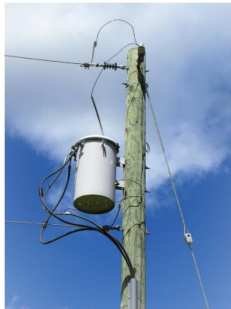
Fig. 4.1: Transformer integrated at a utility pole (source: [pxhere.com](http://pxhere.com), public domain)
